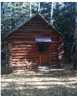
Log Cabin campsite at Camp Westover Lake.
